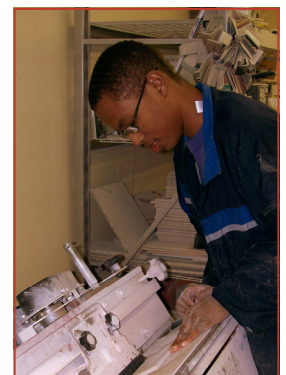
Sheldon cuts and cleans tiles to prepare them for installation.
